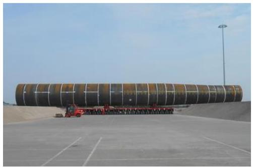
Figure 73: Monopile stored on earth embankments
