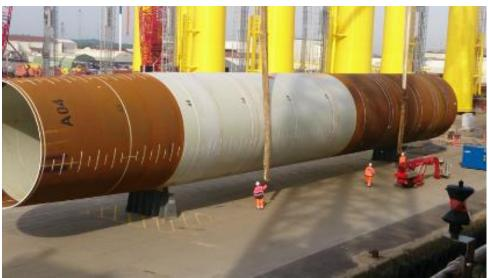
Figure 72: Monopile foundation on steel cradles prepared for loadout
