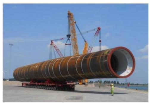
Figure 68: Transportation of monopiles with SPMT
