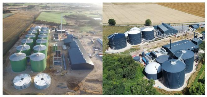
Figure 8 SBS Kliplev (to the left) is approx. 8.5 ha and has an annual production of 48 million Nm<sup>3</sup> of biomethane, whereas Solrød biogas (to the right) is approx. 2 ha and has an annual production of 11 million Nm<sup>3</sup> biomethane [23, 21]
