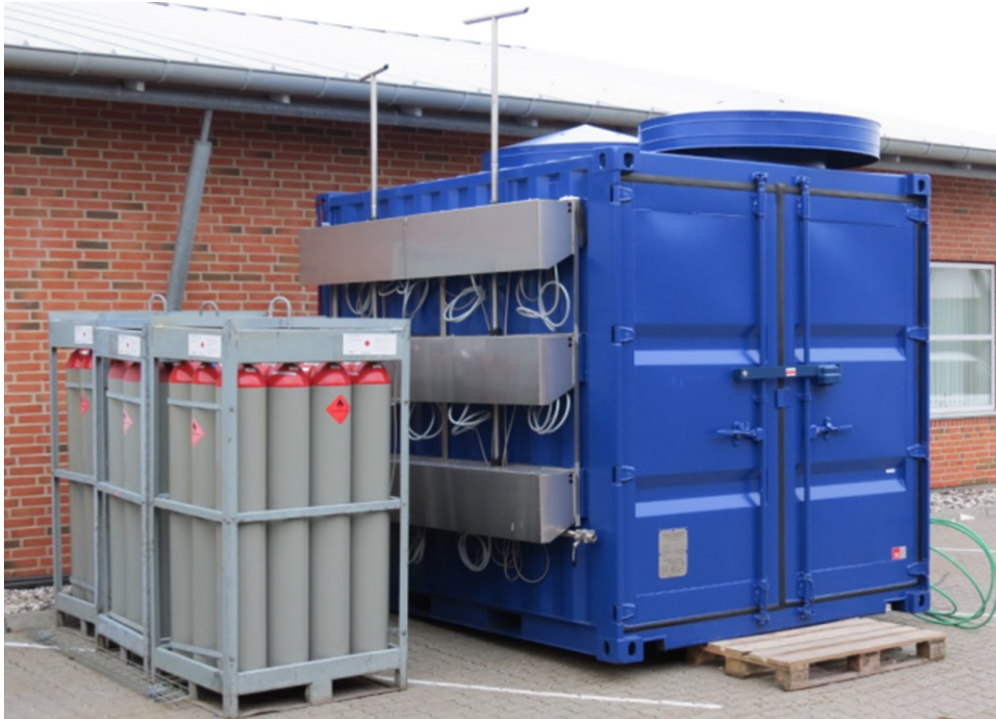
Figure 2: A 50 kW LT-PEMFC CHP hydrogen unit from Dantherm Power.
