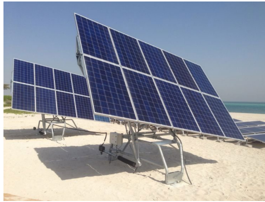
Figure 6 A Helioslite 1.5 tracking system (Ref. 13).
