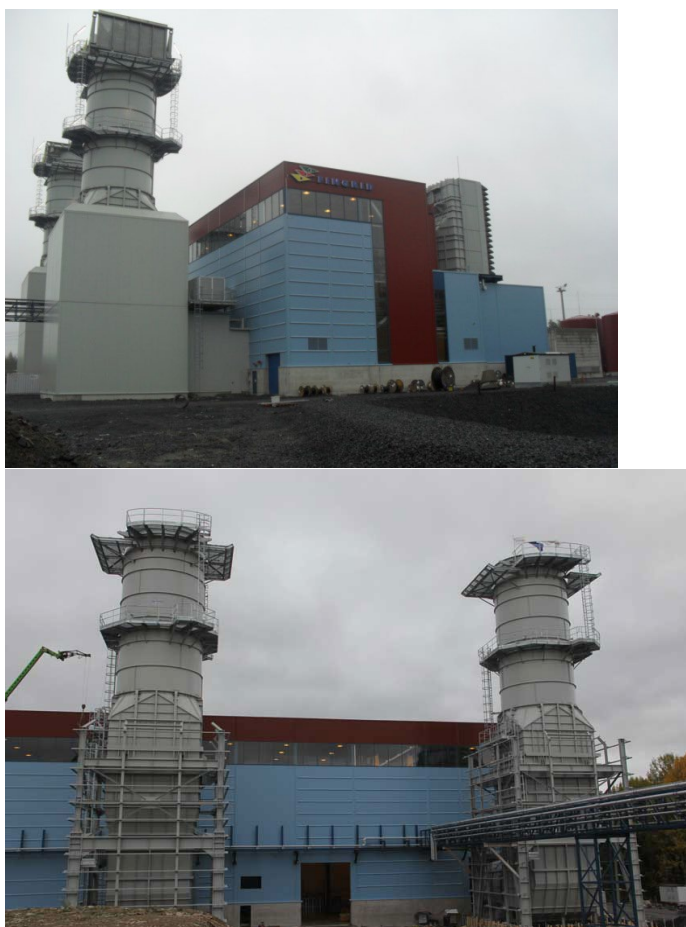
Figure 3 Forssa Power plant commissioned for Fingrid [17].
