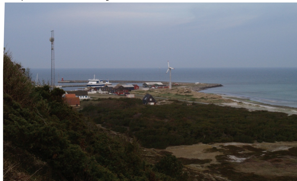
Figure 2-5 View point 1 - Anholt harbour (north)
