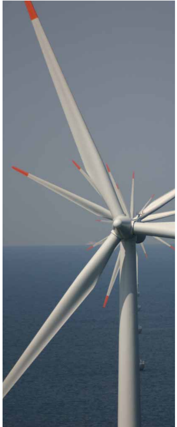
PHOTO: NYSTED OFFSHORE WIND FARM
