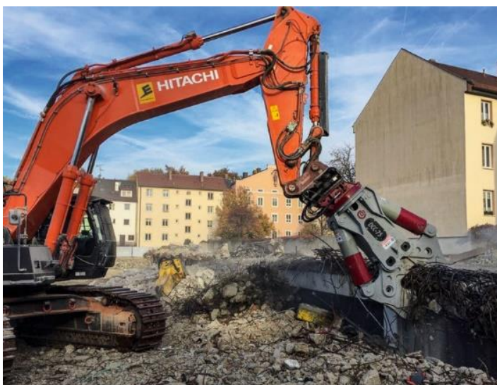
Figure 4 Crusher jaws
